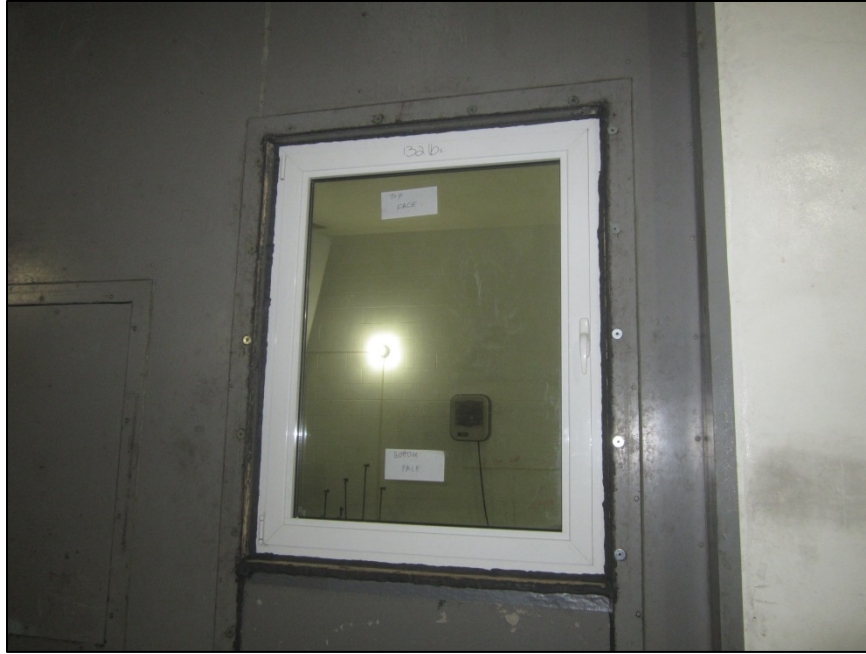
Receive Room View of Installed Test Specimen
